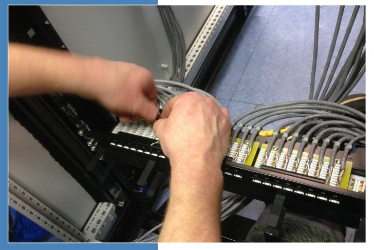
Installing Prefab cabling CAT6 in network and performance check
